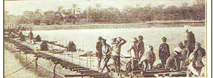
The British engineers constructing a floating bridge across the Tigris. The bridge is built with logs and is being used to transport supplies.
